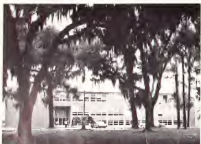
B. F. Hubert Technical Sciences Building.
