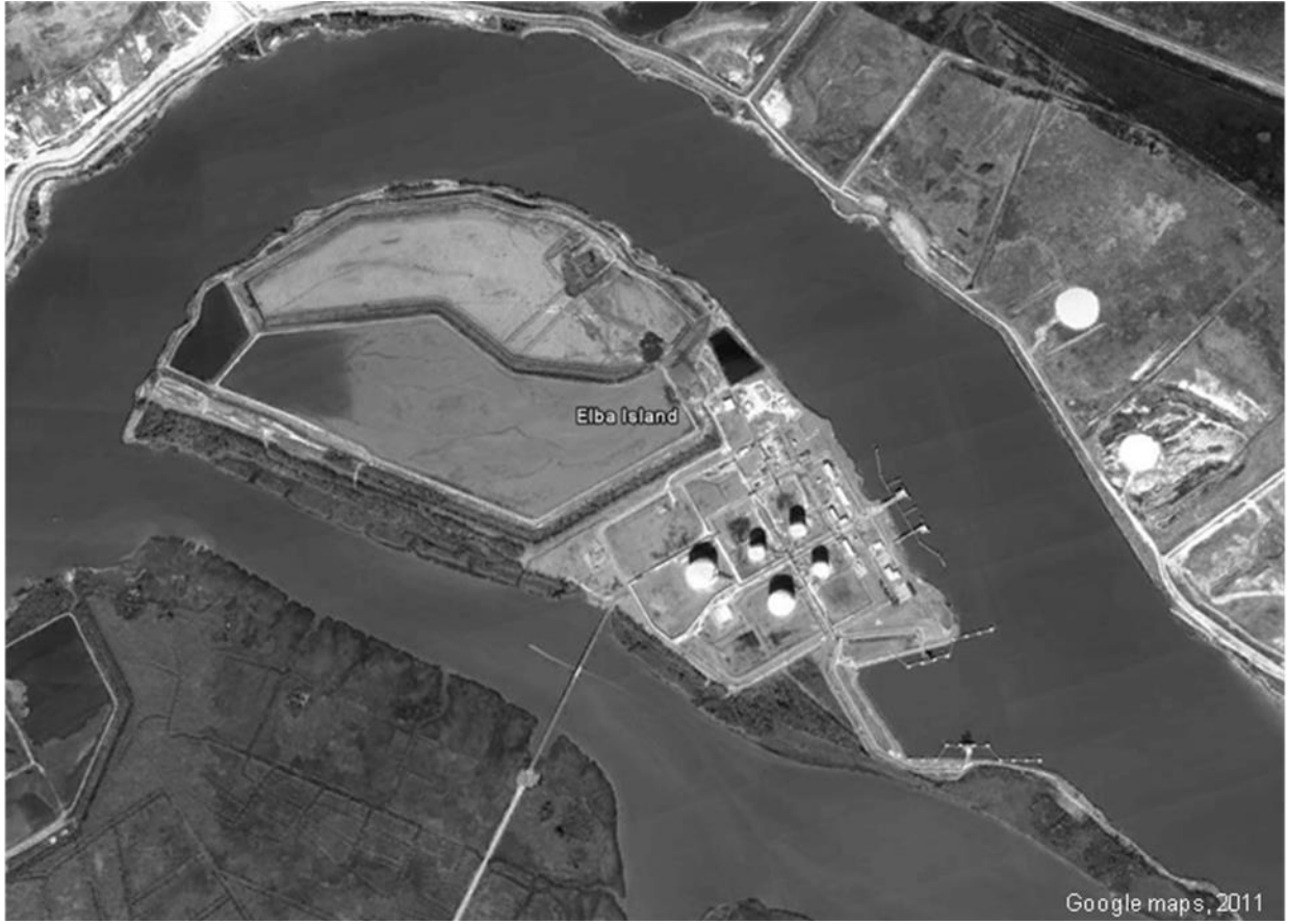
Figure 1. Overhead view of the SLNG regasification facility on Elba Island, Savannah, Georgia.
